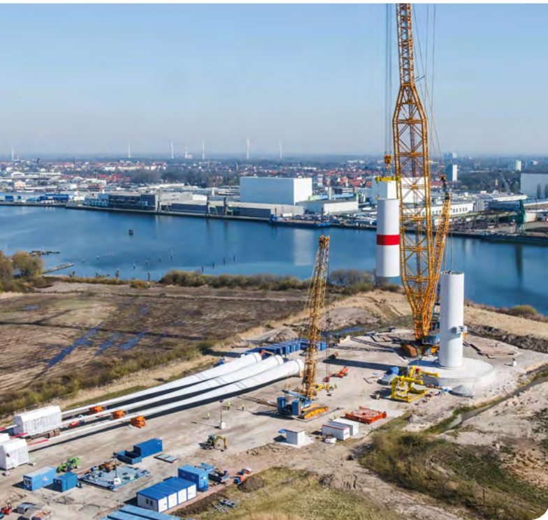
To simplify access, the research facility for testing offshore wind turbines is located inshore. © Adwen
